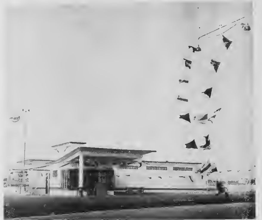
Nerve center for the new aircraft hydrant refueling system is Lago's Aviation Service Building at Dakota Field, gayly decorated for the occasion.
